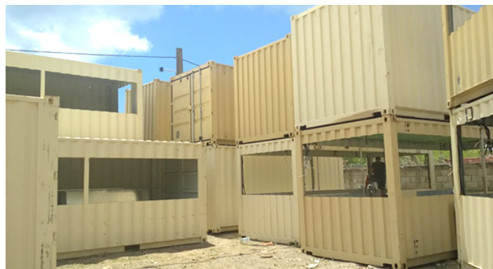
The containers in the process of transformation
