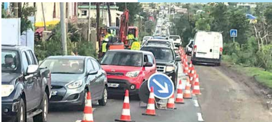
A temporary third lane on the road at La Savane
