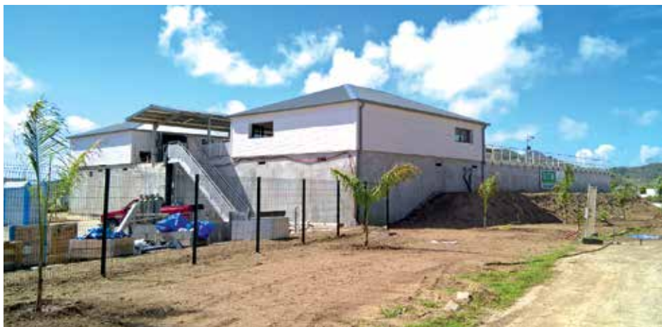
Overall view of the water treatment plant in the French Quarter
